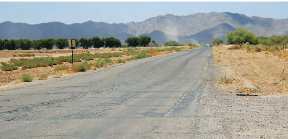
Farrell Road, the main thoroughfare that runs east-west through Ak-Chin Indian Community, shows deterioration from overuse and flooding.
